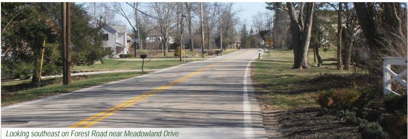
Looking northwest on Forest Road near existing sidewalk
